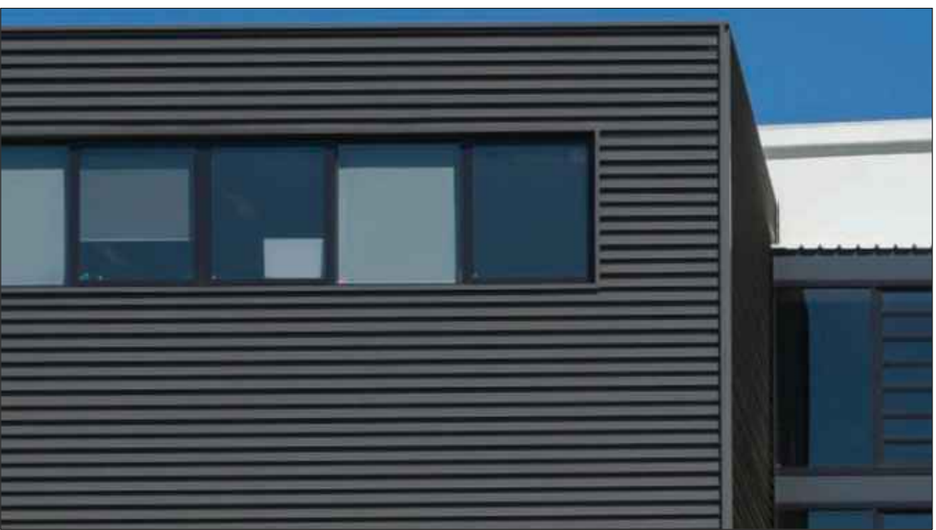
LYSAGHT SPANDEK HORIZONTALLY LAID
